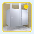
"Floating" or celling hung partitions should be avoided as their original install position will substantially shift over time.
