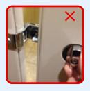
Avoid pre-installed embed latches (most powder coated metal partitions).
